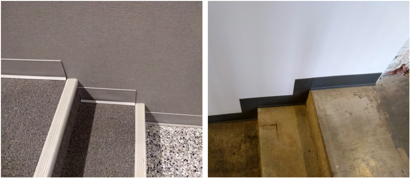
Figure 4. Found conditions—standard detail meets steps. Credit: author.
